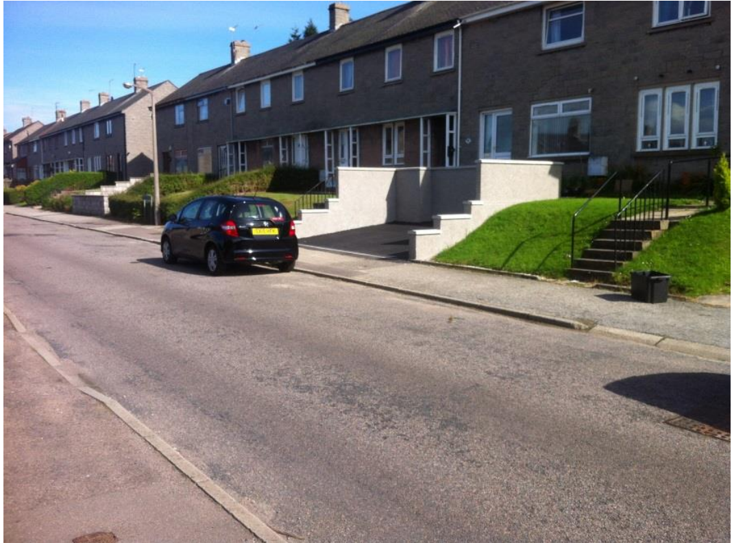
Driveway and retaining walls.
